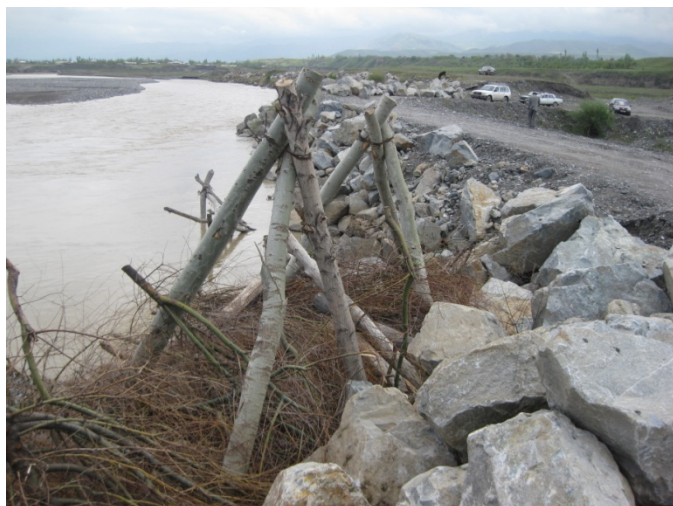
Reinforcement 1 st dam through transport of large rocks from Zeravshan Gold Mine
