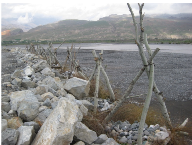
Reinforcement 2 nd dam through transport of large rocks from Zeravshan Gold Mine
