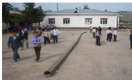
Photo 2 Water pipeline displaced
