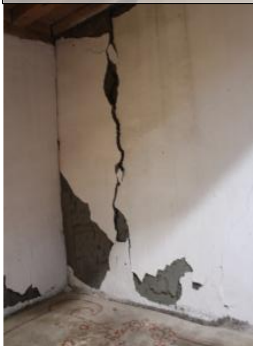
Typical vertical and horizontal cracks, Basid, Tajikistan
