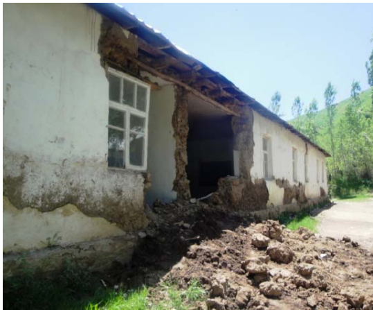
Damage to school #5, Nurabad District
